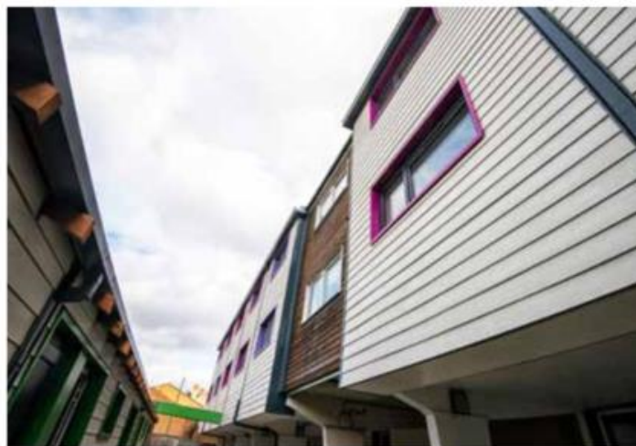
Nottingham City Homes: Energiesprong Retrofit, Melius Homes
